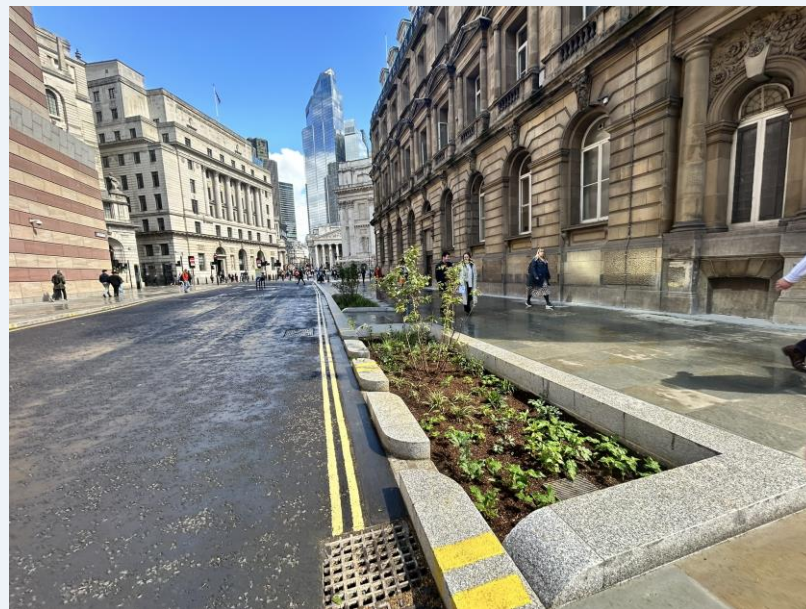
Bank Junction 'rain gardens' completed Apr 2024, full greening due to be completed Sep 2024.
