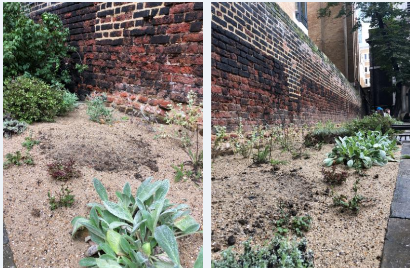
All Hallows by the wall sand beds completed in Spring 2023.
