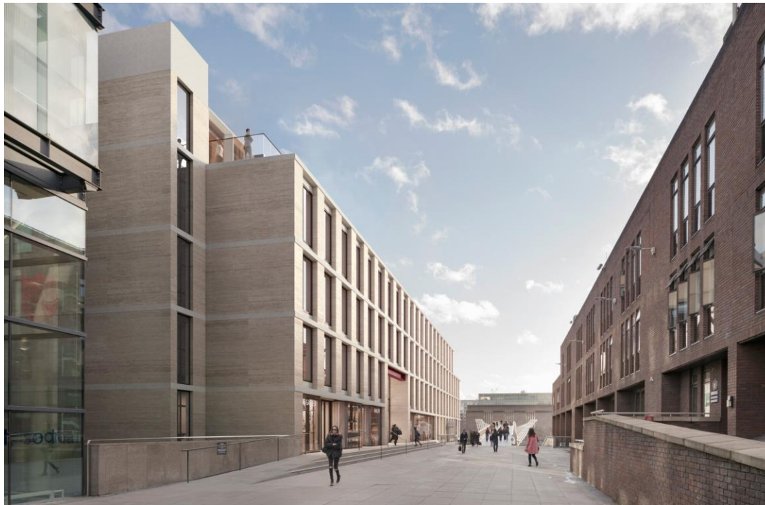
Millennium Bridge House photomontage of completed development, looking south to the Bridge
